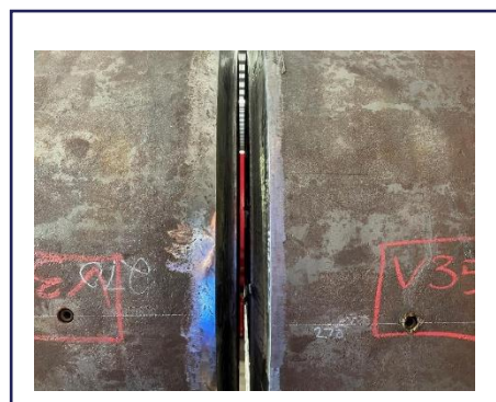
Figure 19: Re-welding of the reactor shell.
