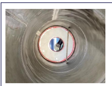
Figure 18: Installation of the new liner.
