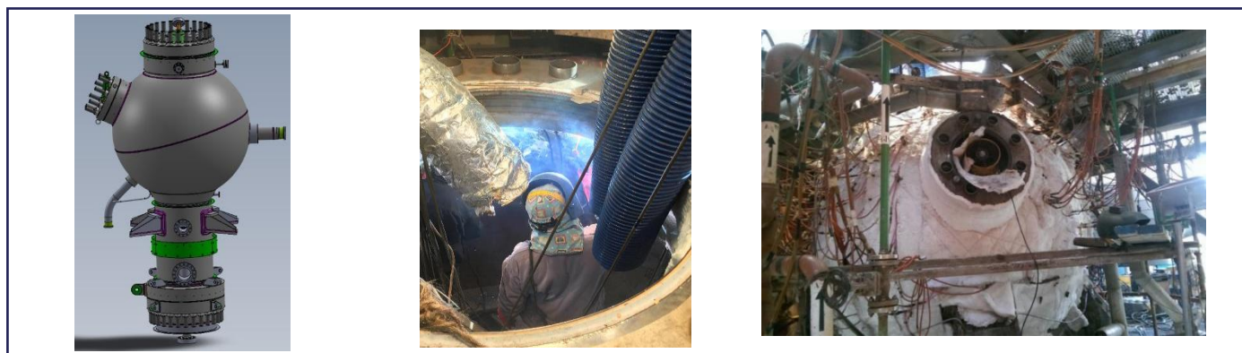
Figure 4: Repair of damaged sphere of the HP scrubber at Abu Qir, Egypt.
