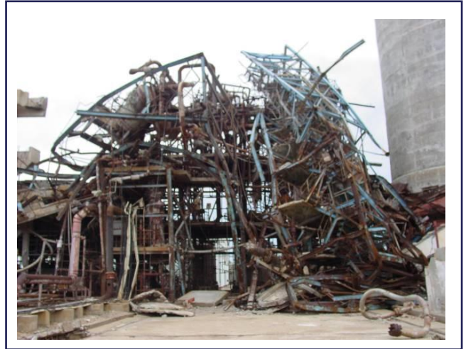
Figure 2: Catastrophic failure of a urea reactor destroying a urea plant.
